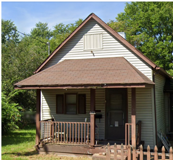
503 Walter Jetton before
