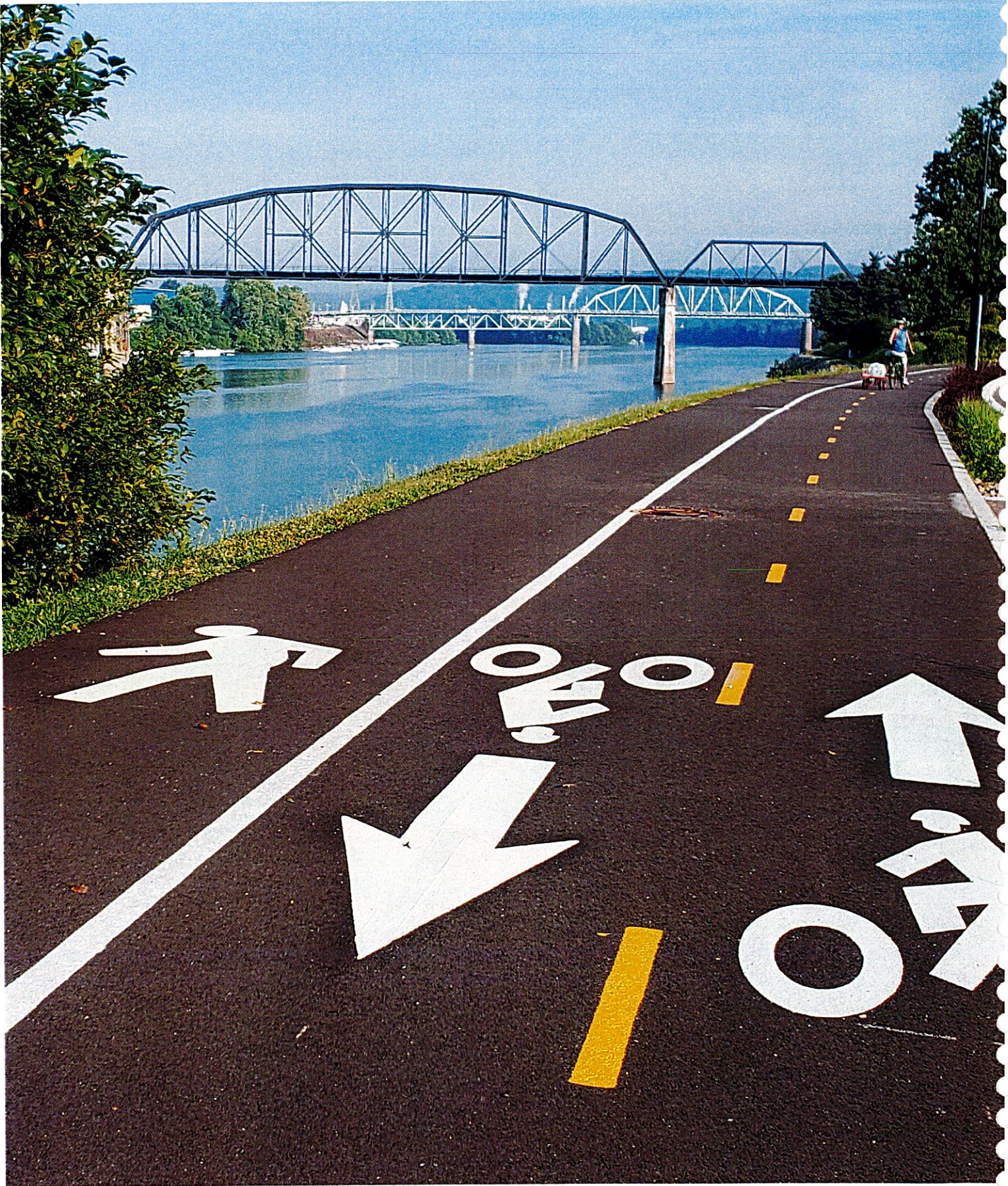
^ Kanawha Boulevard Bikeway | Charleston, West Virginia
