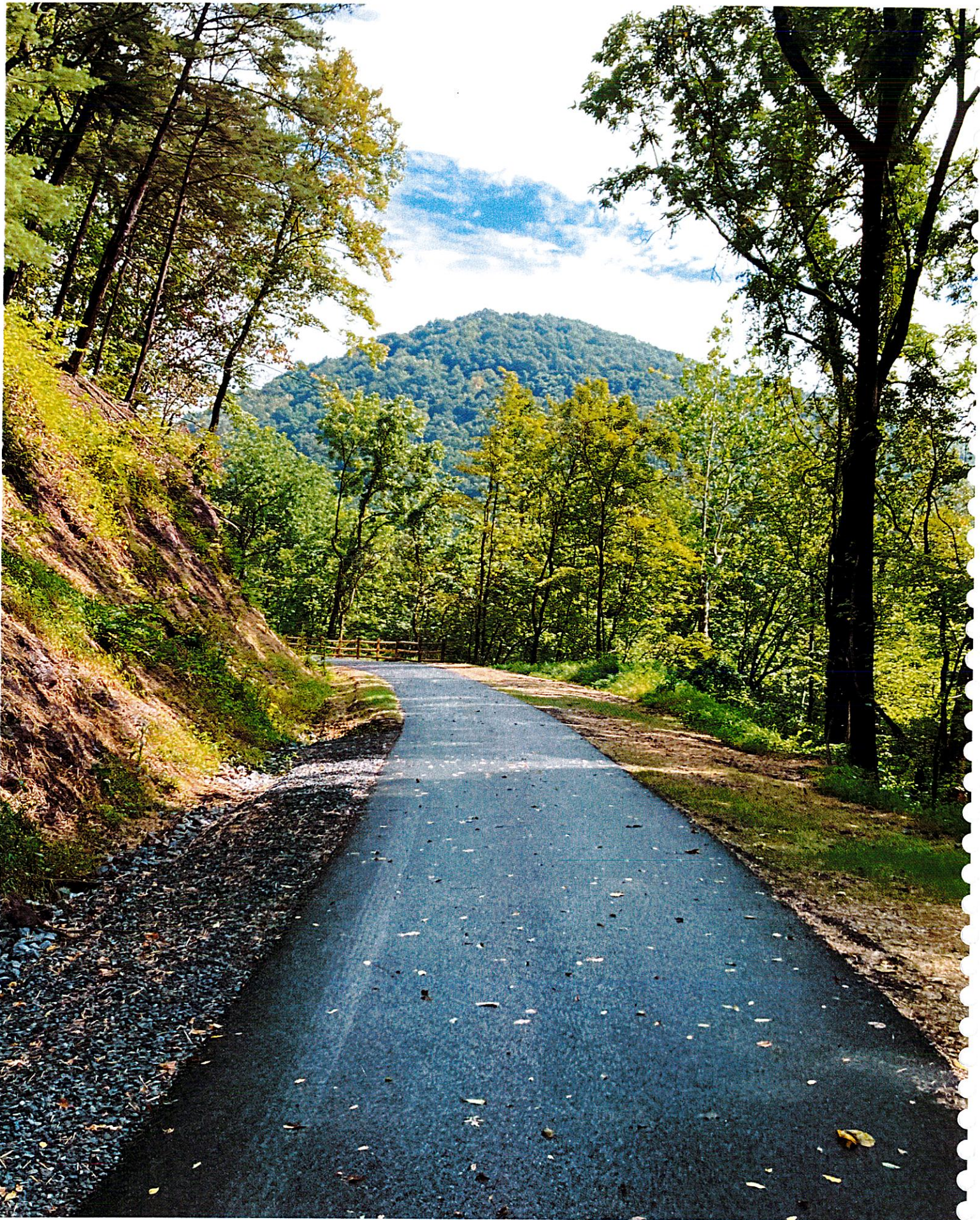
^ Huntington and Broad Top (H&BT) Trail Design and Engineering | Broad Top Township, Pennsylvania
