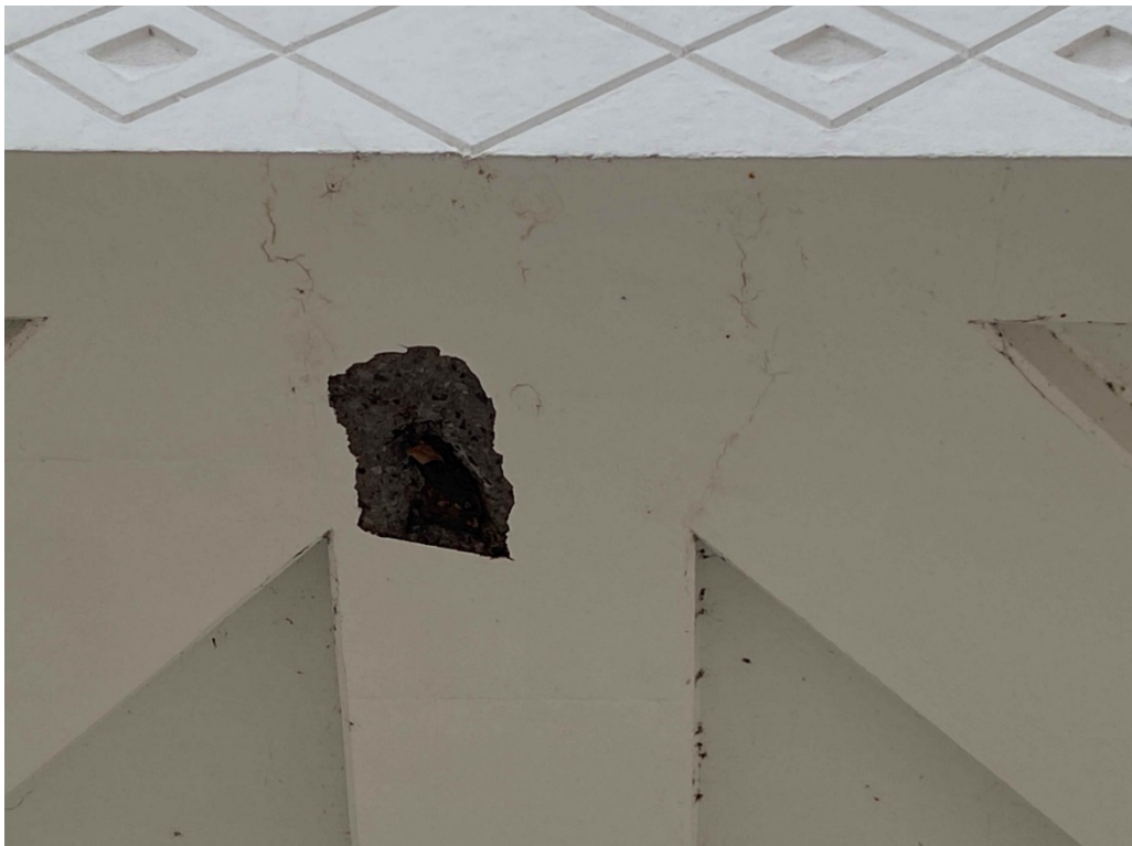
Photo 2 (Spalled Portion)
