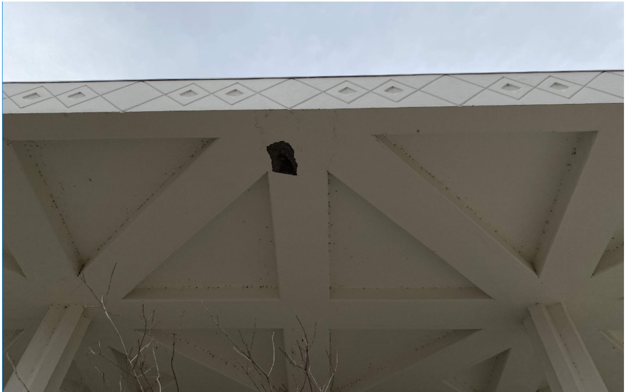
Photo 2 (Spalled Portion)
