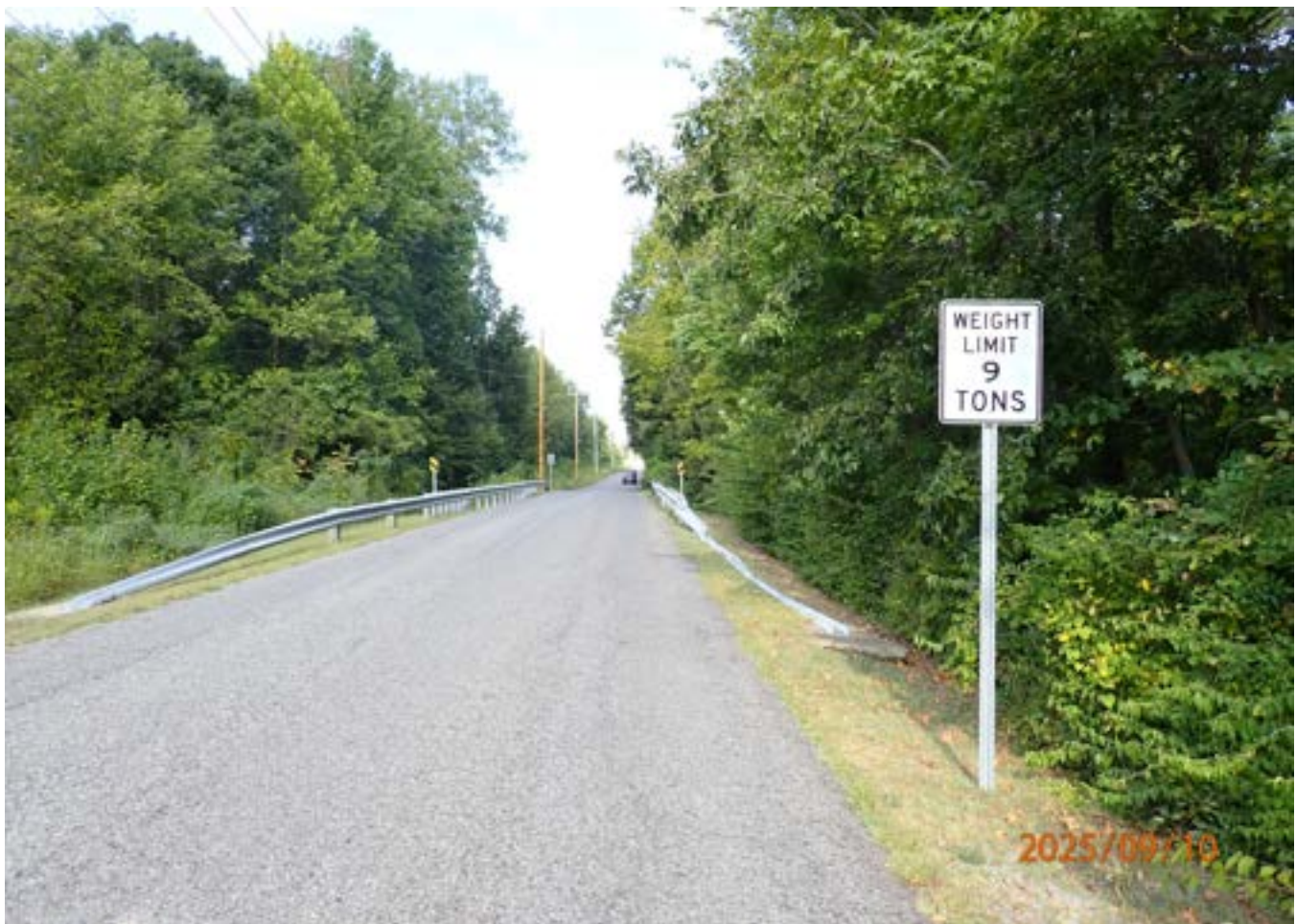
Looking west - posted sign in place
