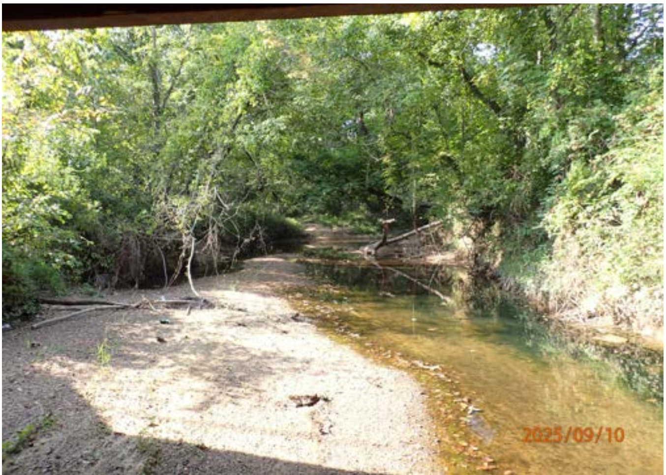
Looking upstream from under bridge
