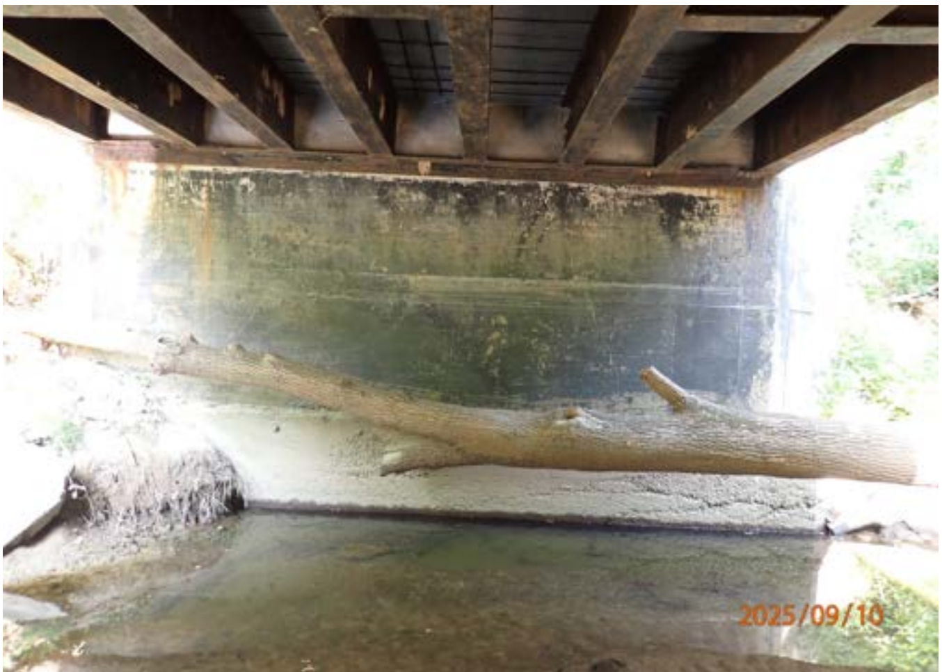
Abutment 1 - footer exposed
