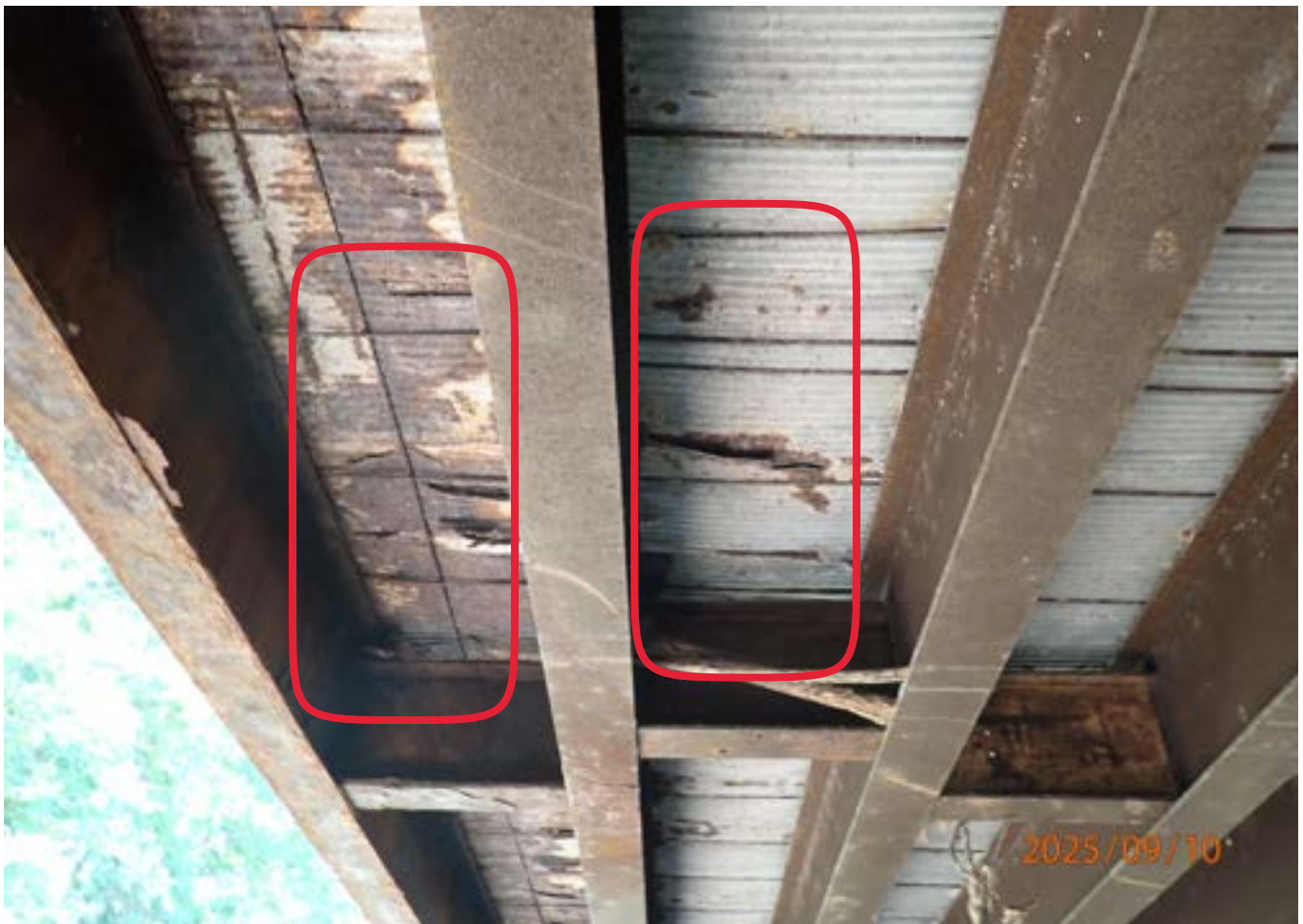
Typical of metal stay in place forms
