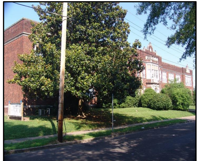
Looking northeast into the site
