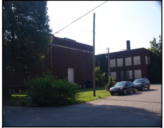
Looking northeast into the site
