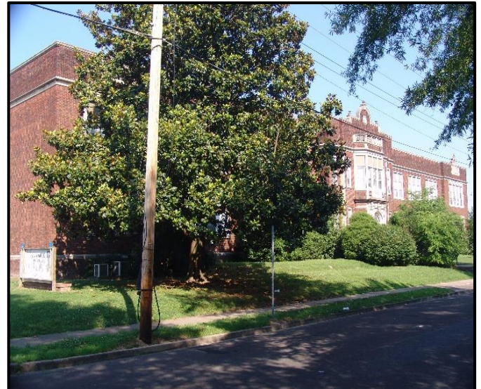
Looking northeast into the site
